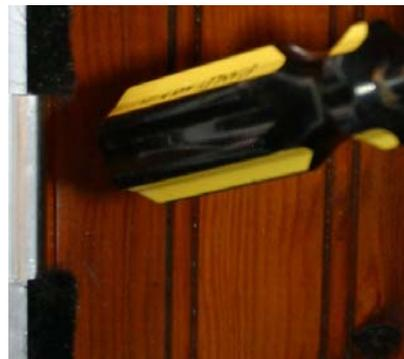
Carefully tap on magnets to adjust downwards.
