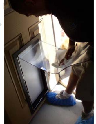
You may also adjust the magnets in the frame if necessary. They can either be raised or lowered so the flaps seal but swing freely. Adjust the magnets upward by twisting a flat headed screwdriver below the magnet between the magnet and the frame. Adjust the magnets downward by tapping lightly with the handle of your screwdriver.
