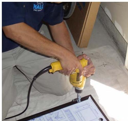
**Step 9:** Put the inner frame of the pet door (the one with the security cover track) into the rough opening in the people door. Slide the outside frame into the other side of the door and let the pet door frame sleeve together. Squeeze the two sides of the pet door frame together tightly.
